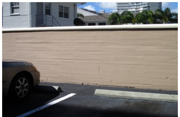
32 Perimeter Wall Overview
